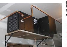
A. Connect cooling water inlet and outlet pipes to cooling water source. Closed loop cooling tower, lake water, or geothermal water source systems are recommended.
