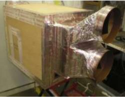
6. Completely seal all seams, top, bottom, front back and both sides with foil tape. Do not cover the drain line or the electrical outlet on the condenser side.
